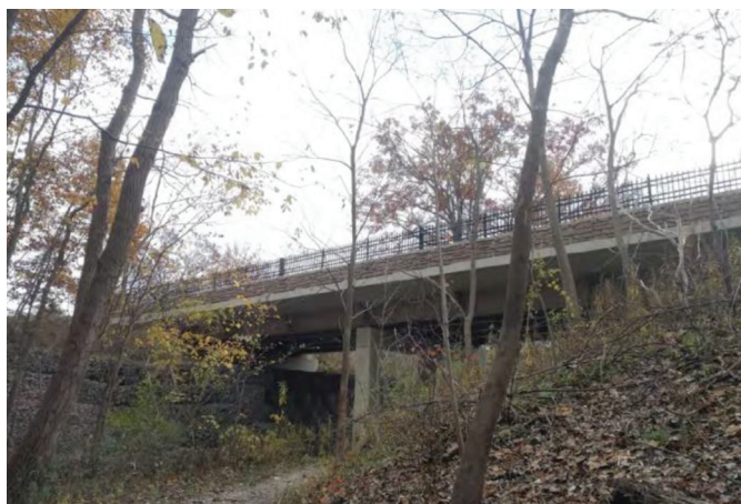
Fig. 2 Cuyahoga County Bridge (Miles Road Bridge No. 178) – deck entirely reinforced with GFRP rebars (Benzecry et al., 2019)
