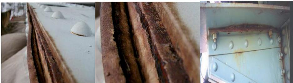
*Fig. 2. Crevice corrosion on steel elements [21]*
