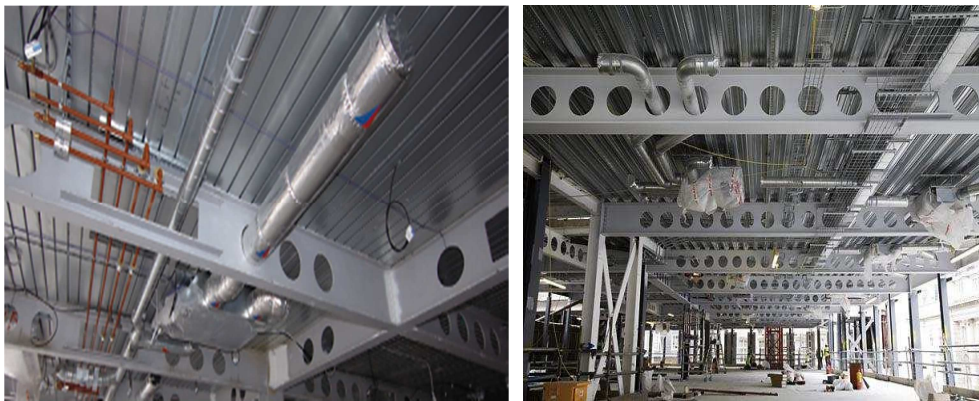
Fig. 3: Web opening in frames.
